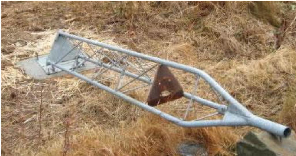
Recycling a basketball hoop base, which provides built-in height and stability, is another alternative the tower option has.
